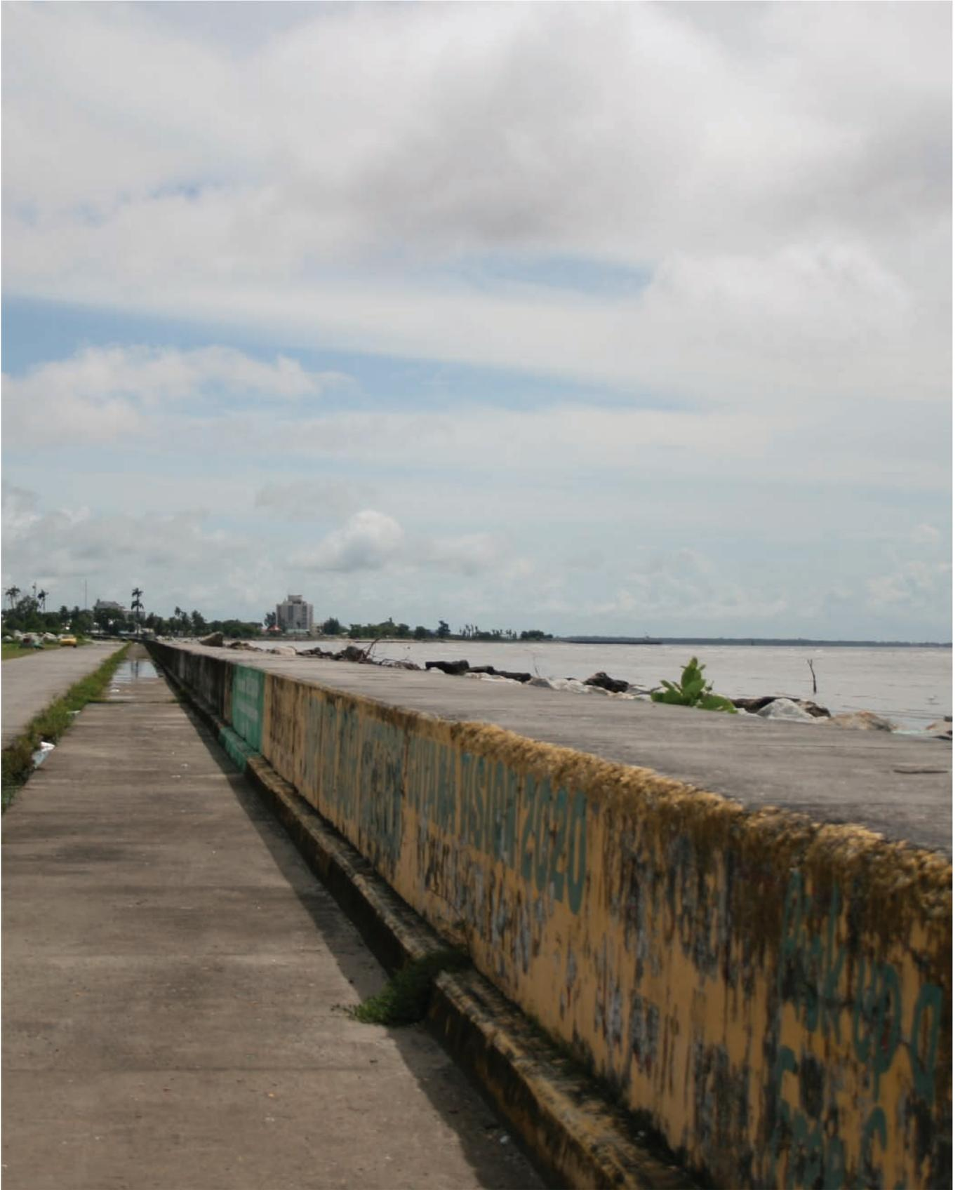
Seawall, Georgetown, Guyana. The seawall was built along the foreshore to protect low-lying coastal areas from flooding
